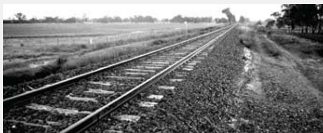
Seed spilling from trains (and trucks) is the major source of volunteer canola.
