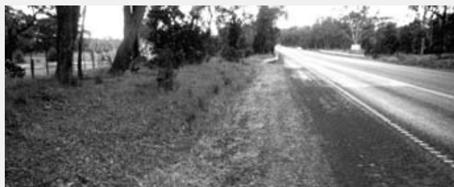
A narrow strip of verge sprayed with Roundup to prevent damage to the bitumen, saves slashing costs and improve drainage.
