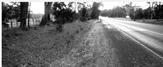
A narrow strip of verge sprayed with Roundup to prevent damage to the bitumen, saves slashing costs and improve drainage.
